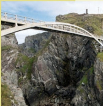
Mizen Head Bridge
